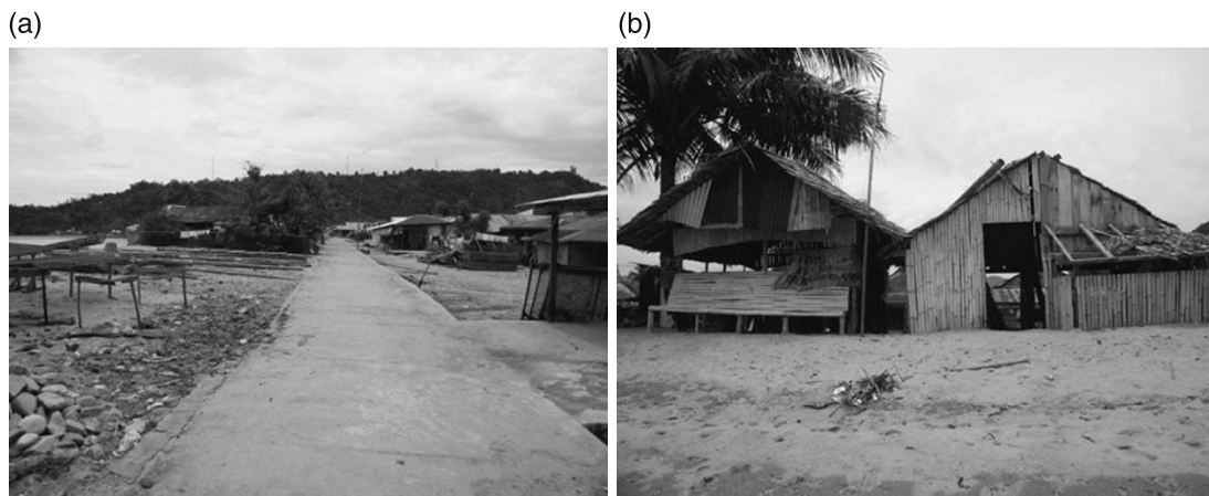
Fig. 6. Houses and the road near the Painan beach. Left: A cement road about 5 m wide approximately parallel to the shoreline. The distance between the shoreline and the road is about 60 m. Right: Wooden houses with iron roofs just behind the high-tide line.
