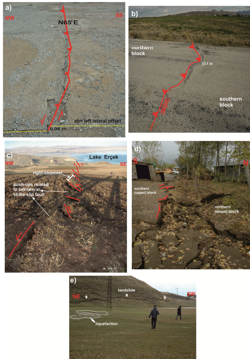
Fig. 3. (a) A view of left-lateral offset on a concrete block, caused by the MSR. (b) A view from the main surface rupture (MSR) on the Topaktaş road. The vertical thrust offset is approximately 0.1 m. (c) The NE-SW trending, left-lateral strike-slip fault surface rupture with transpressional component (push-up structures) on the west side of Lake Erçek. (d) The en-echelon shaped tensional cracks in Erciş. (e) View of the landslide and liquefactions near Topaktaş village.
