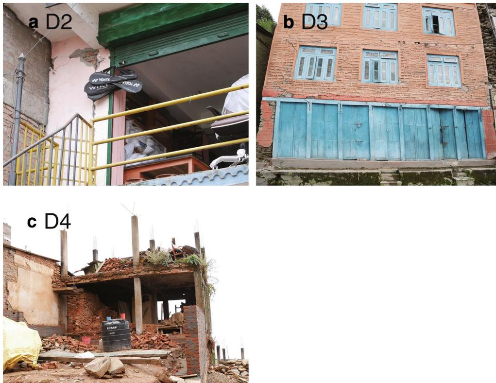
**Fig. 4** Photograph of buildings with damage levels D2–D4. **a** D2: plaster on the column was fallen down. **b** D3: permanent drift was observed. **c** D4: almost all infill was fallen down
